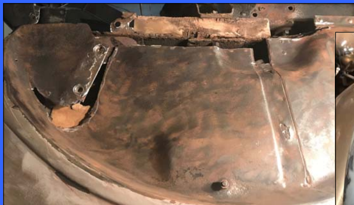
Well panel with rust-out removed.
