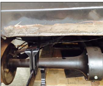
Photo 9: Rear deck welded and ready for glass finish.
