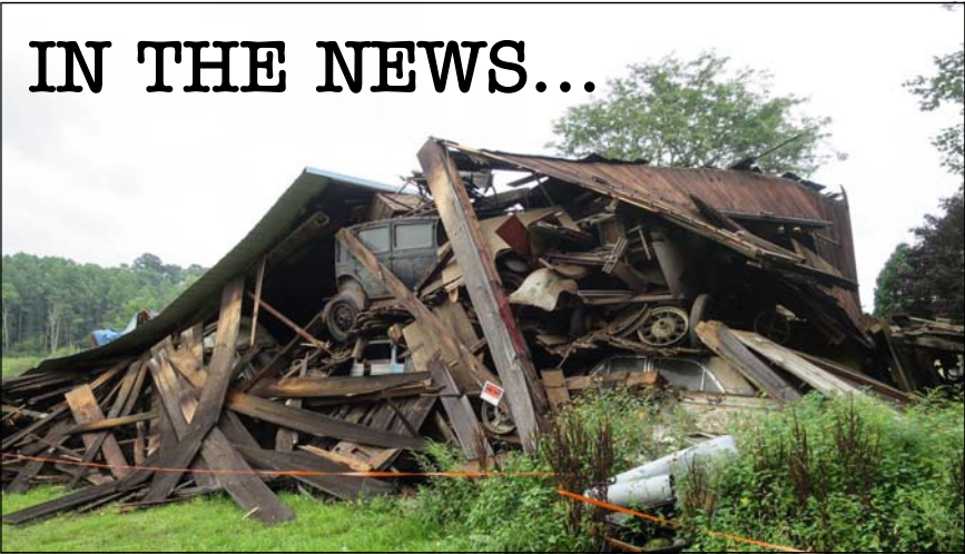
Tragic Pennsylvania Barn Collapse
